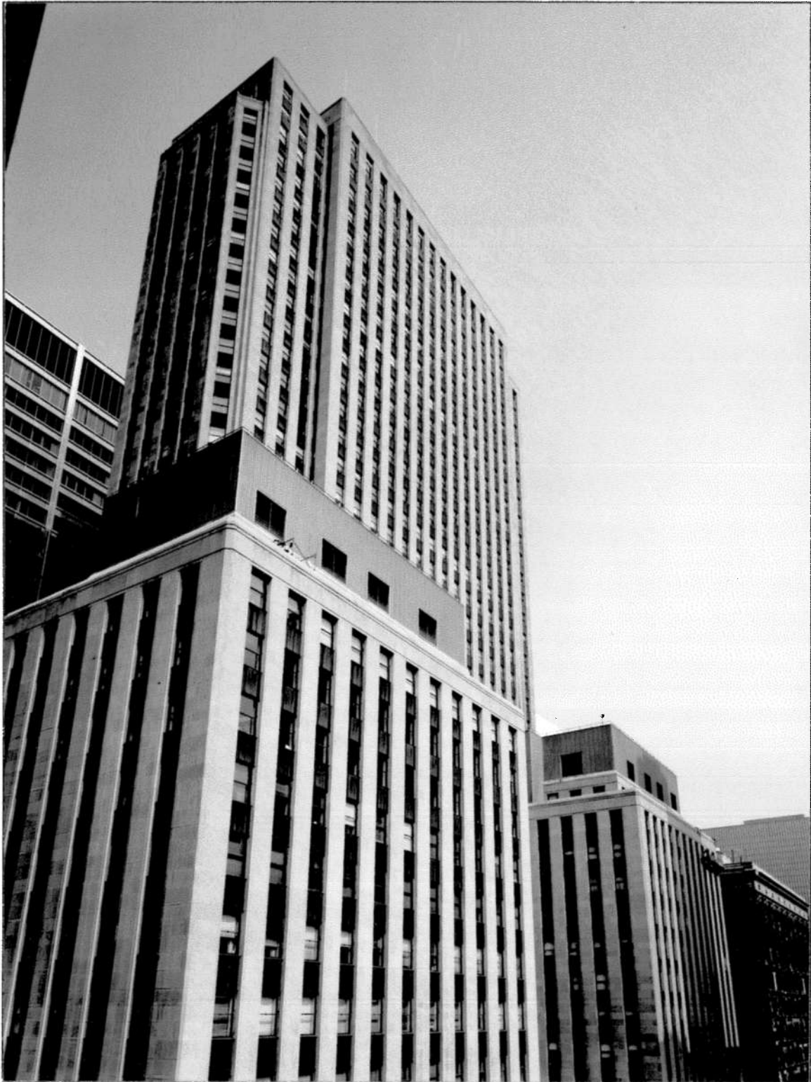
Chamfered corners sculpt the forty-three-story central tower and twenty-two-story surrounding wings of the limestone clad Field Building. (Bob Thall, photographer)
